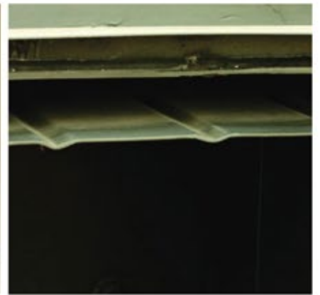
Bypass system automatically opens when you open the door to stop smoke leaking out.
